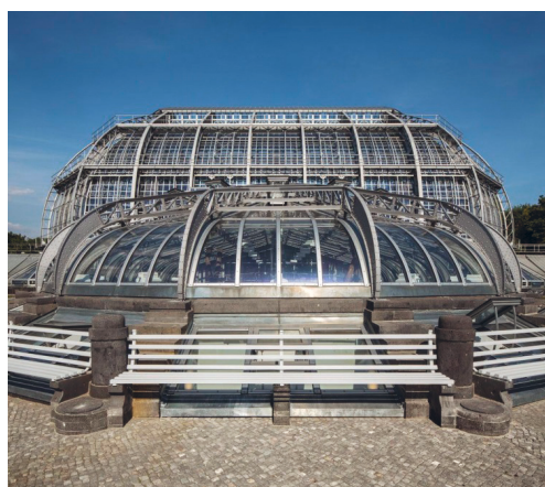
Figure 1. Large Tropical Conservatory after the renovation, Victoria House in the front (Photo: Dirk Altenkirch).
