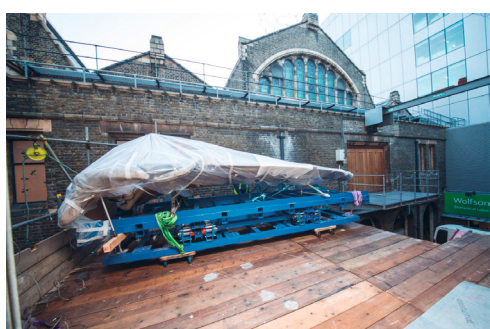
Figure 8. Due to the complex and high-risk nature of removing the whale skull, it required a specialist frame for support.
